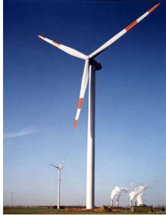
Figure 1.1 Nordex N80 2.5 MW turbine 80m Tower 80m Rotor Diameter
